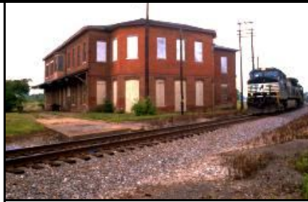
Pre-fire view of the Union Station with a train passing on the NS Railway, and the CSX Transportation line abandoned across the station's front
